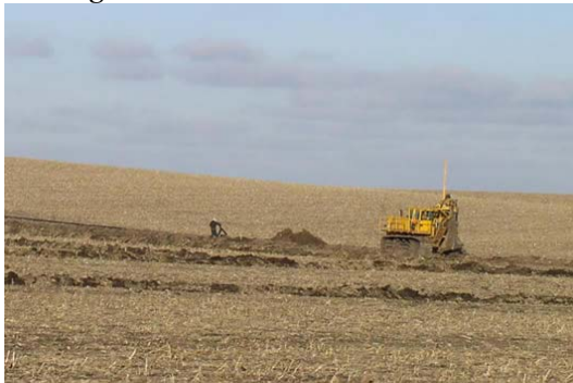
Tile installation in the UIRW.
